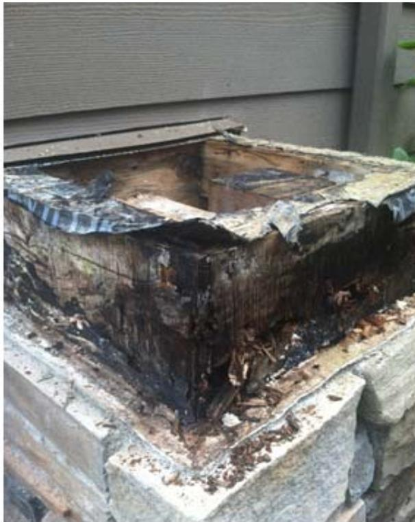
1           82.     As with corbels and knee braces, Shea replaced failed columns on its own model
