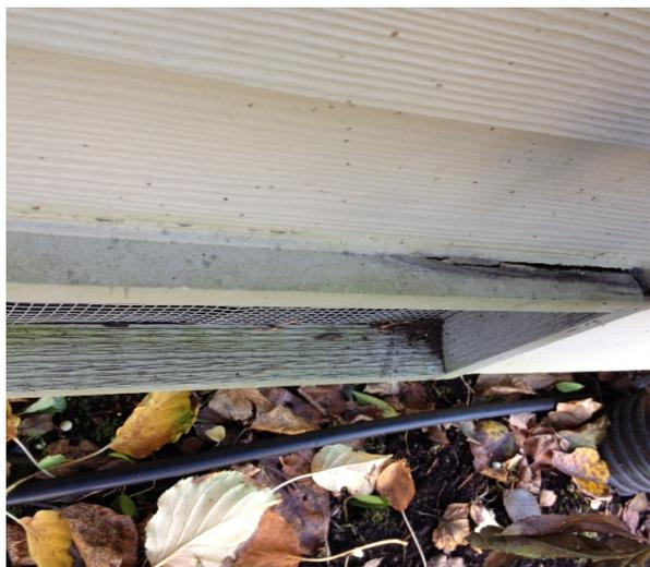
27           148. Shea also failed to install an adequate number of vents on many homes. And even
