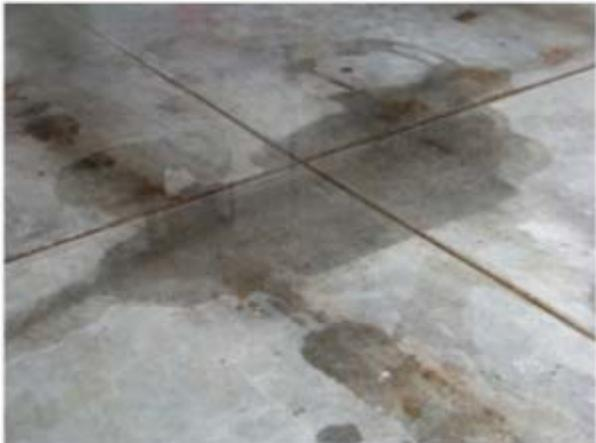
44. Even at houses where Shea attempted to conceal the problem by installing plastic tiles on top of the wet garage floor before selling the home, evidence of the problem is now apparent as efflorescence makes its way up through the joints in the plastic tiles:
