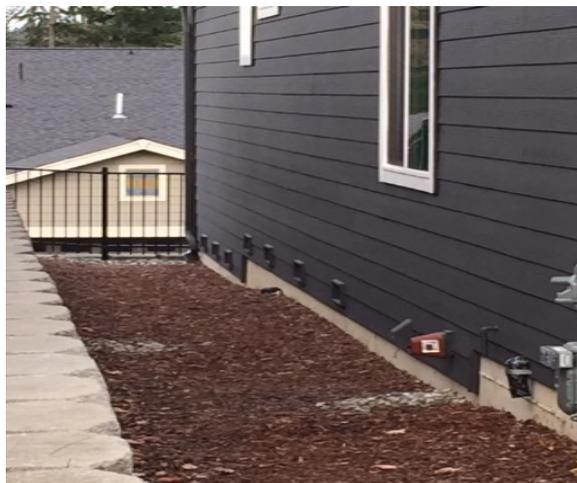
13 The above photograph shows crawlspace vents along just one elevation of at recently built
