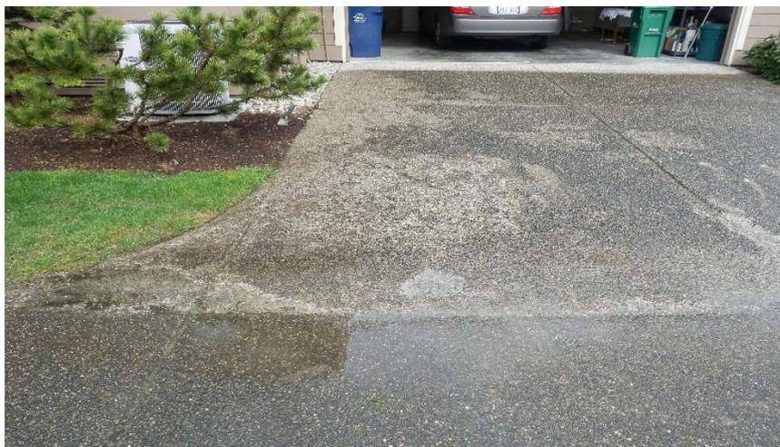
20 121. The failing, spalling driveways built by Shea lead to pooling water and further
